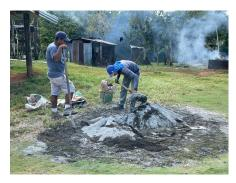
Well #91: For the Los Corrales extended family system, the Agua Viva Serves team mixed and poured concrete around the well casing to prevent water from entering the top of the well; laid out, dug, formed the re-bar and poured concrete for the tower footers: .8x .8x 1 meter deep (lots of digging and mixing). The family will put a fence around the well to keep their livestock away from the well head.
